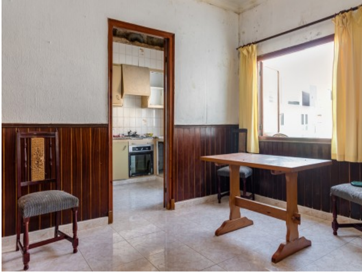
The town house needs a renovation
